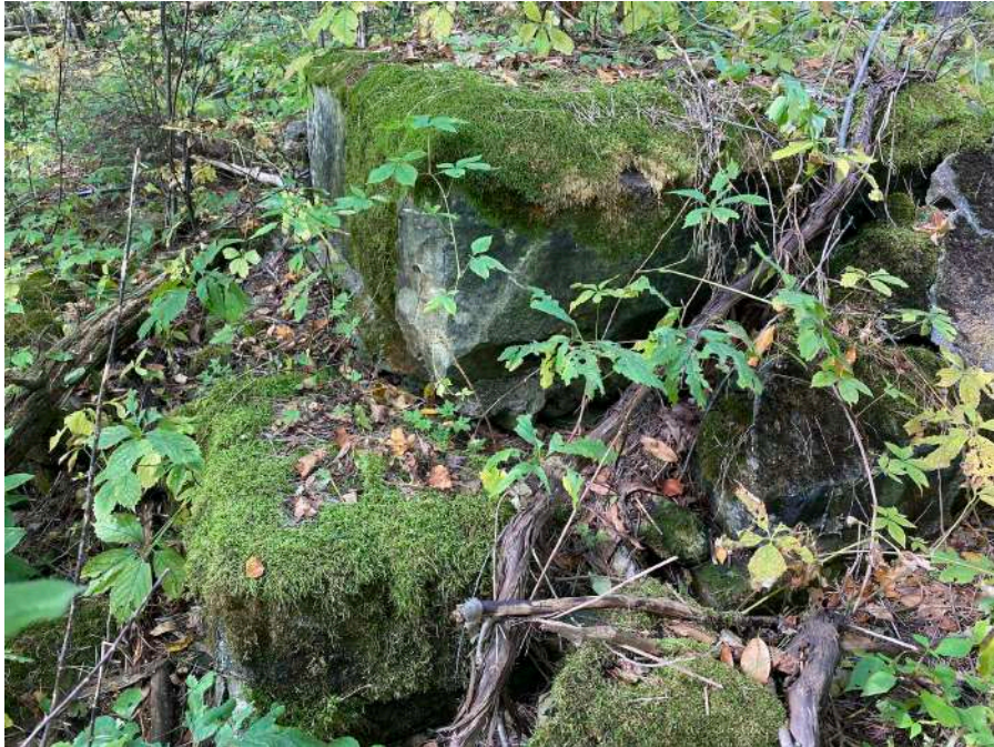
Image 15. Southwest foundation block of former railway water tank showing deterioration of the stone blocks and concrete. View to the west.
