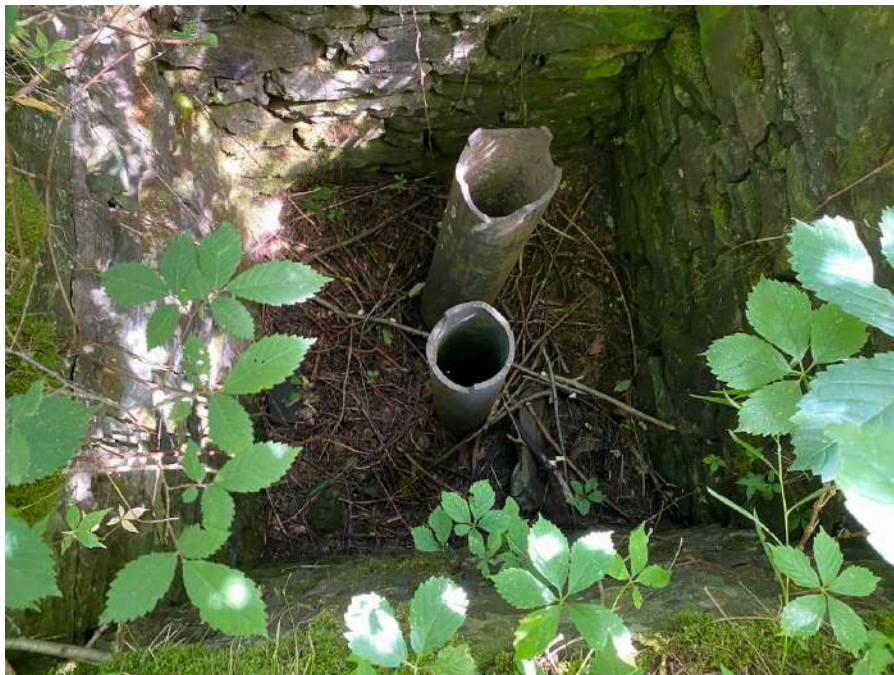
Image 17. Centre well of former railway water tank.
