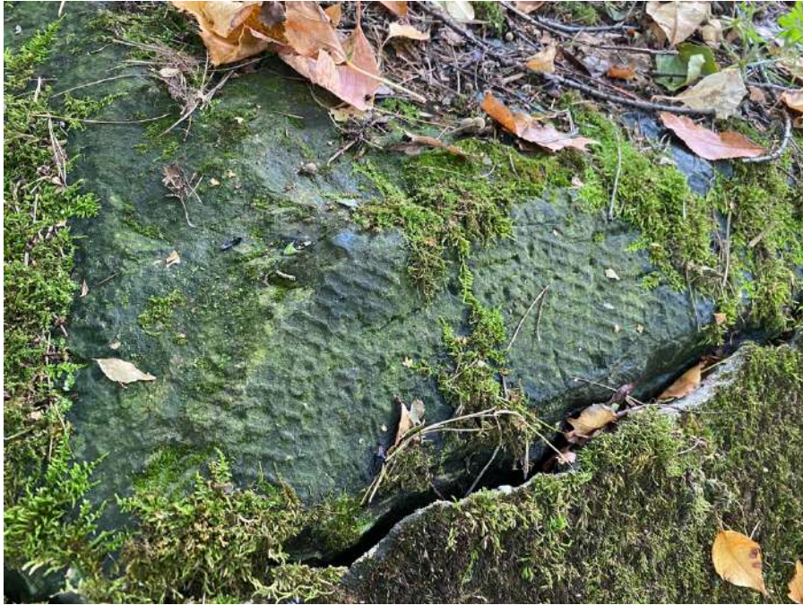
Image 13. Southeast foundation block of former railway water tank showing stone dressing and concrete.
