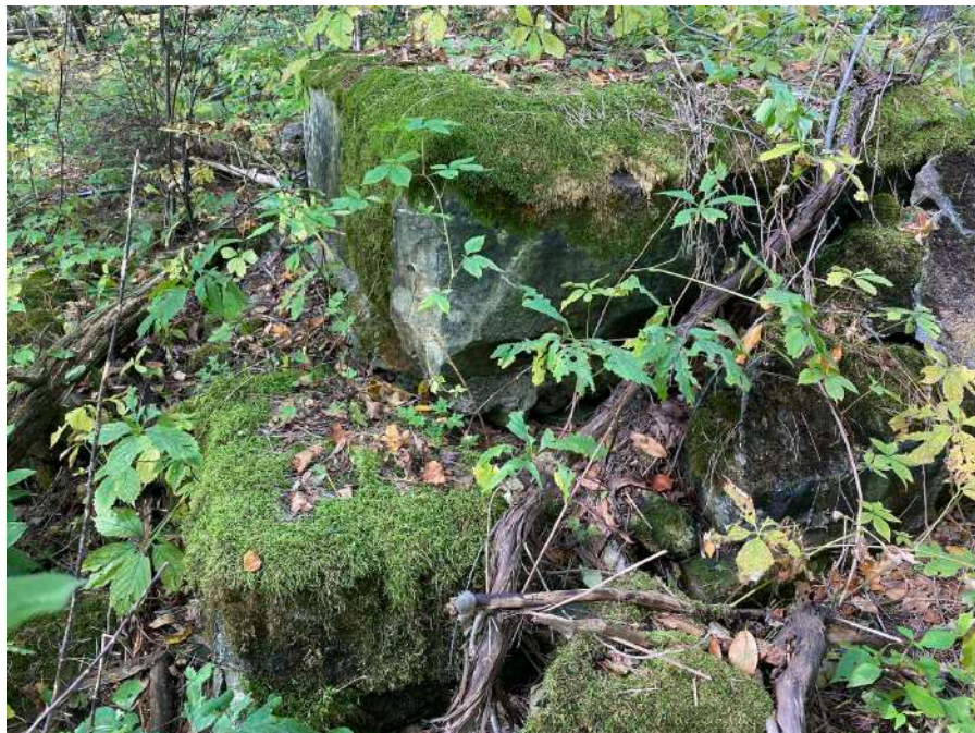
Image 15. Southwest foundation block of water tank showing deterioration of the stone blocks and concrete. View to the west.
