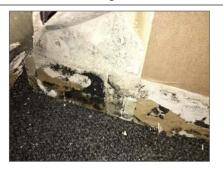
Photo 4 – Mould growth on the concealed side of the wallpaper and north drywall wall.
