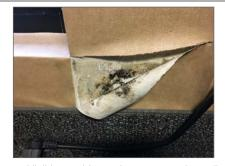
Photo 3 – Visible mould growth present on the wall paper and east drywall wall.
